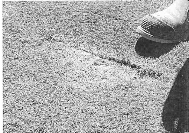
Depressed area / possible trip hazard requiring practical stabilization.
