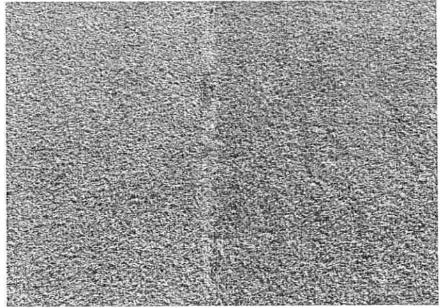
Visible seam wear and surface separation through turf fibers.
